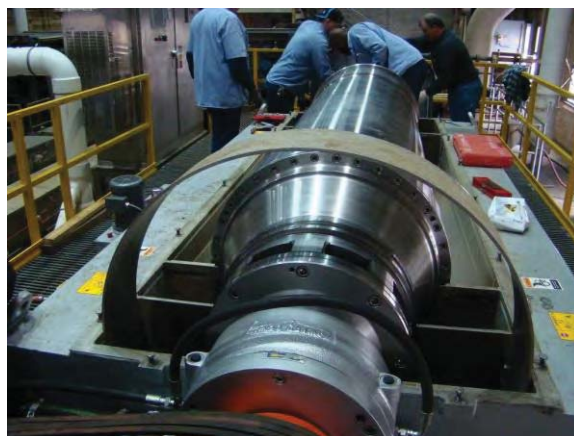
Maintenance staff from the Facilities Management Division troubleshoot sludge dewatering equipment at the Downriver Wastewater Treatment Facility
