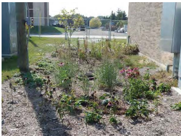
"Grow Zone" established by the Water Quality Management and Facilities Management Divisions to filter storm water from the Marter Road Booster Pump Station, Northeast Sewage Disposal System
