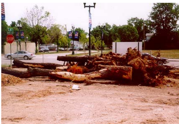
Trees removed for construction are a resource, woody debris for instream structure.
