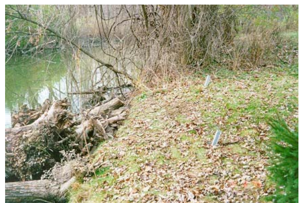
Logs are affixed to the bank by cables and stakes. This activity requires a MDEQ permit for installation.
