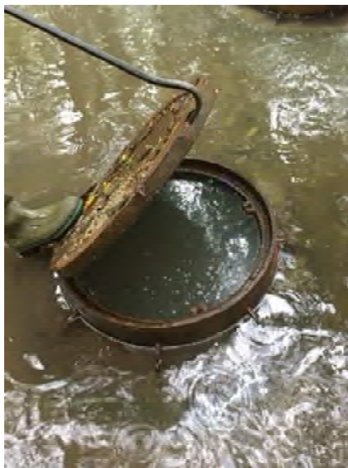
Figure 4-1: Manhole M-20 (Middle Rouge Interceptor) – September 29, 2017; River Level and Interceptor Level Equalized
