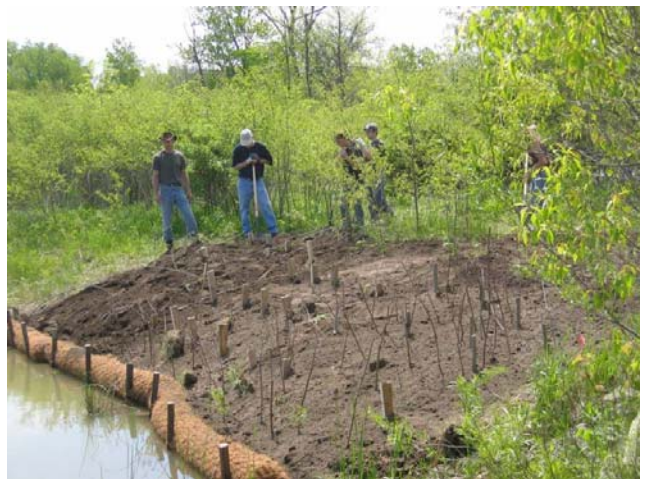
The streambank is stabilized with installed live fascines, live posts and brushmattress (B. Szczechowski)
