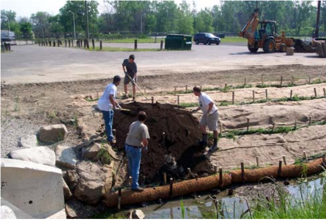
Volunteers cover the fascines with topsoil . (Picture - S. Harbour)
