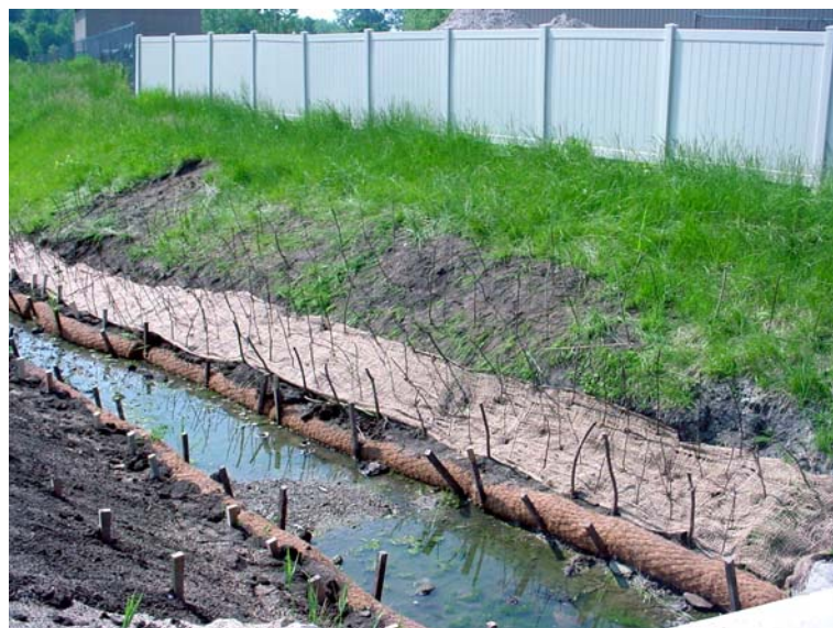
The southern streambank is stabilized with live stakes and native wildflower seed (M. Best)
